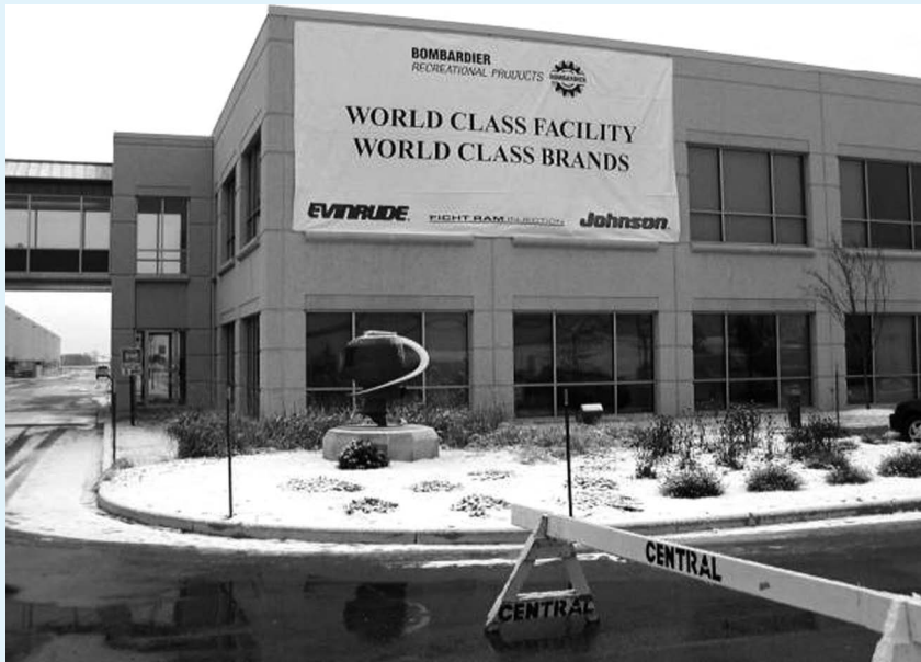
FIGURE 4-21 NEW EVINRUDE-JOHNSON PLANT IN STURTEVANT, WISCONSIN
