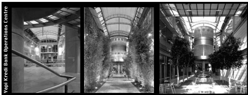
The ten courtyard office buildings are linked by covered courtyards and walkways that imitate the traditional Ottoman marketplaces.
